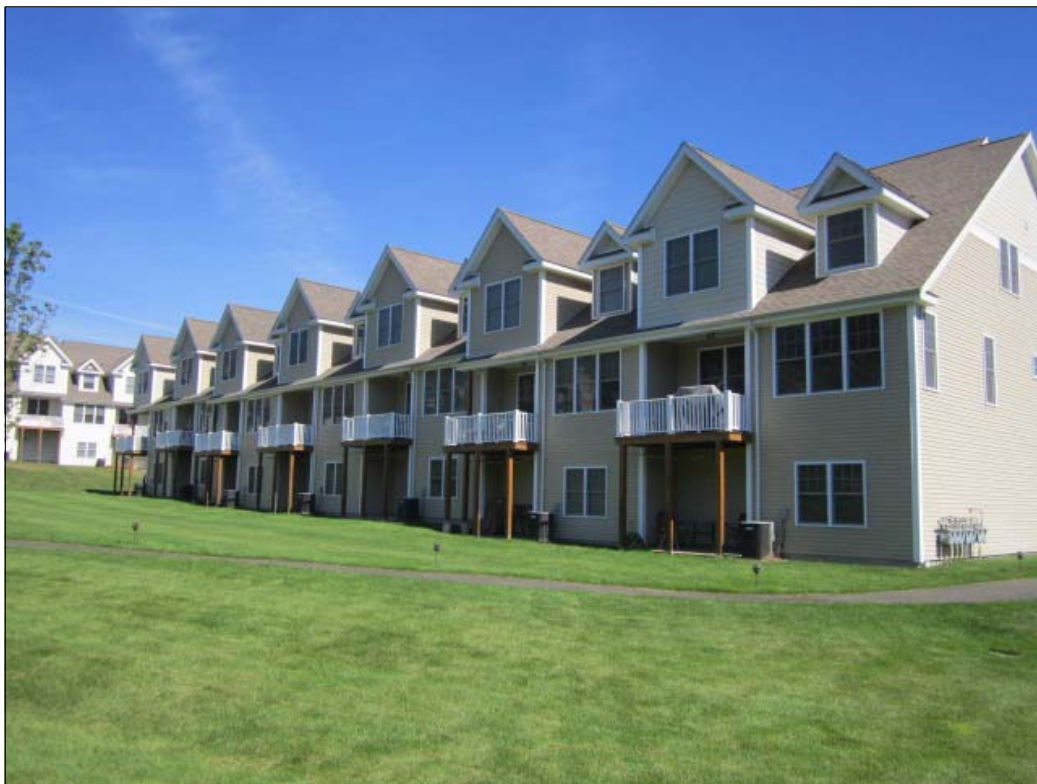
Rear of 7-Unit TH Building
