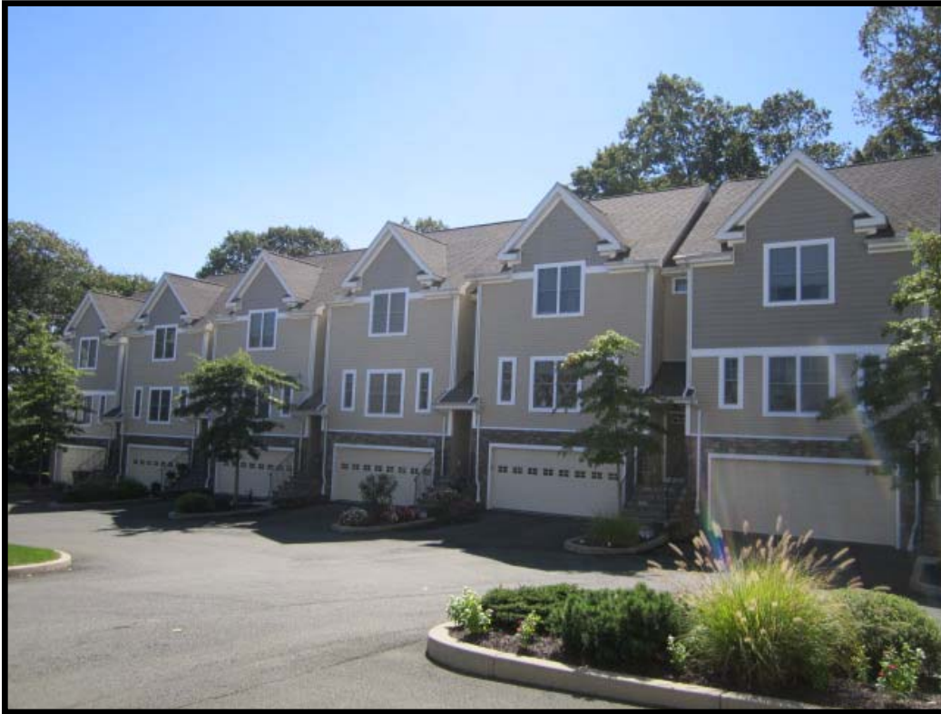
Front of 6-Unit TH Building
